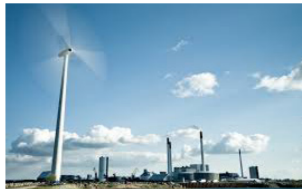
Sustainable biomass and new energy technologies – two of the ingredients for future climate-friendly district heating. Photo by HOFOR.
