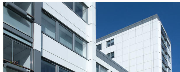
The apartments at Bellmanskade after energy retrofitting. Photo by NCC.
