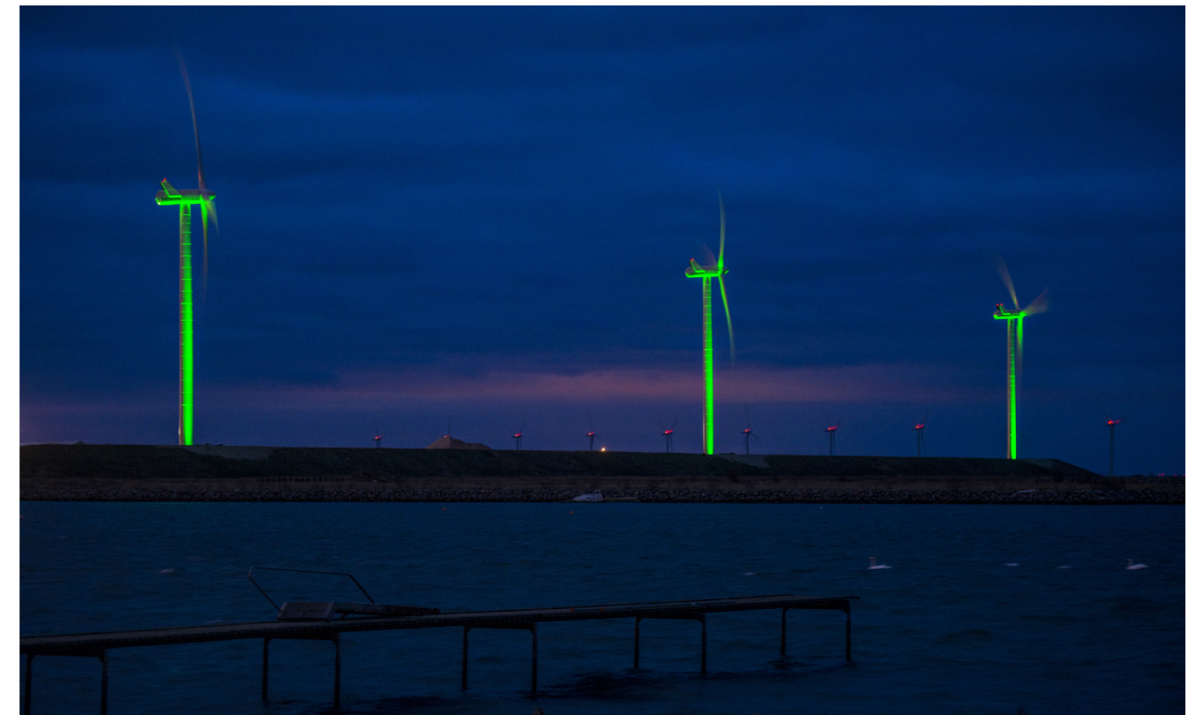
The three new wind turbines at Prøvestenen on the day of their inauguration. Photo by HOFOR.
