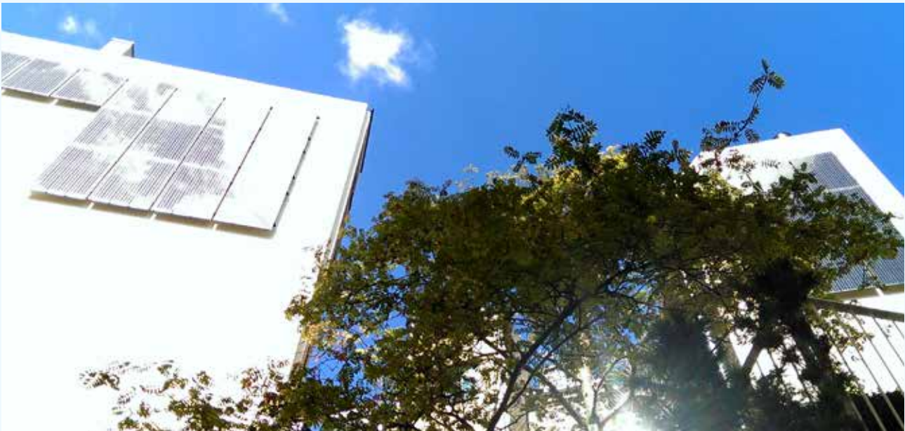
A thorough urban renewal demonstration project, testing new technologies for ventilation and with solar panels on the roof and gables, a green roof and penthouses. Gammel Kongevej 51 / Værnedamsvej 18-20. Photo by City of Copenhagen.
