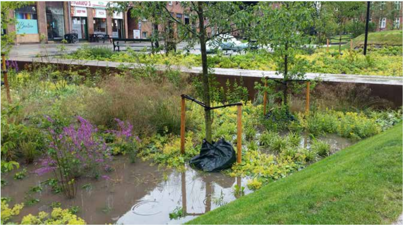
Tåsinge Plads passed the test after its first cloudburst in July 2015. The renovated square is designed to store and divert precipitation away from the neighbourhood. Photo by Mette Fjendbo Petersen.
