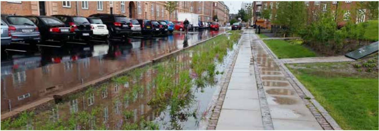
After undergoing major renovation, Tåsinge Plads is ready for cloudbursts. The square now serves as an important element in securing the neighbourhood against climate change by collecting, delaying and seeping precipitation. Photo by Mette Fjendbo Petersen.
