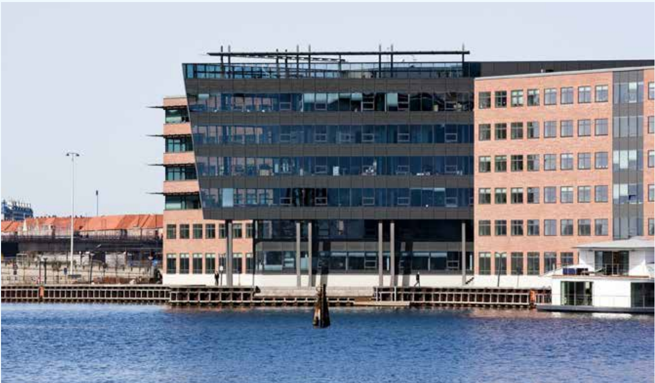
New windows with built-in shading in Norrportens Building, Kalvebod Brygge 45. Photo by Ulf Areskoog.
