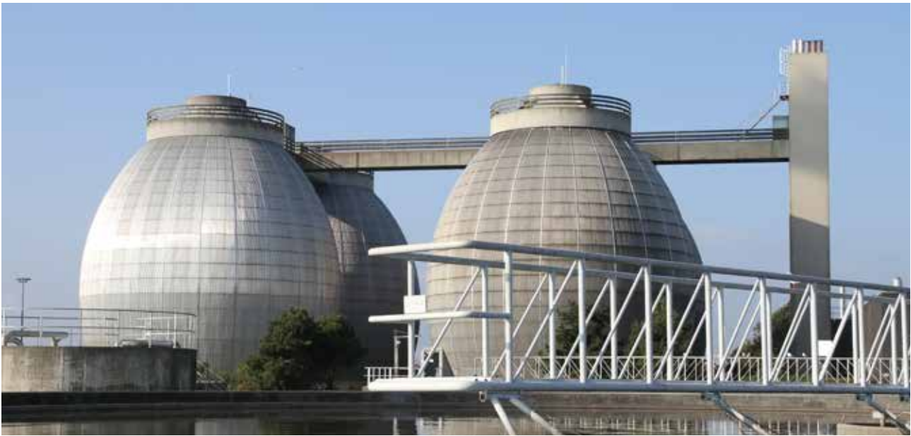
Biogas production in digesters at BIOFOS. Photo by BIOFOS
