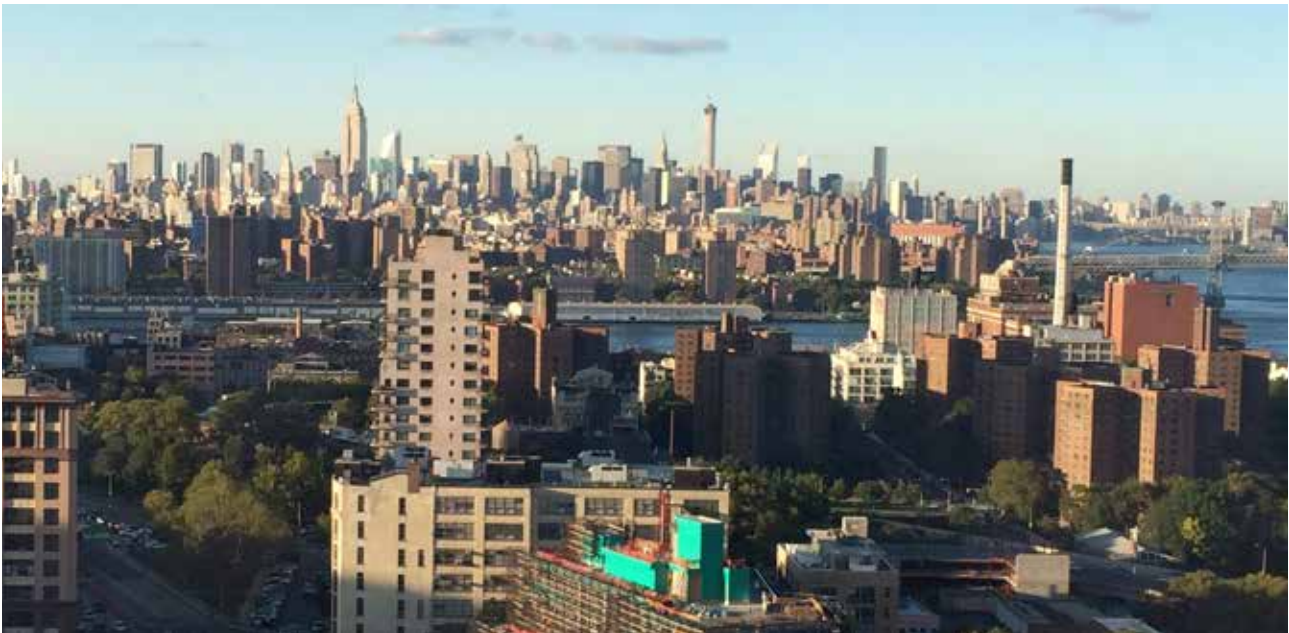
Most of New York's buildings have on-site heat production. Photo by Jørgen Abildgaard, City of Copenhagen
