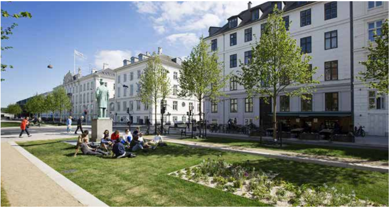
Skt. Annæ Square was designed to handle large amounts of precipitation during cloudbursts by lowering the square so it slants towards the middle instead of towards the edges. Photo by Søren Svendsen/Kvæsthusprojektet.dk
