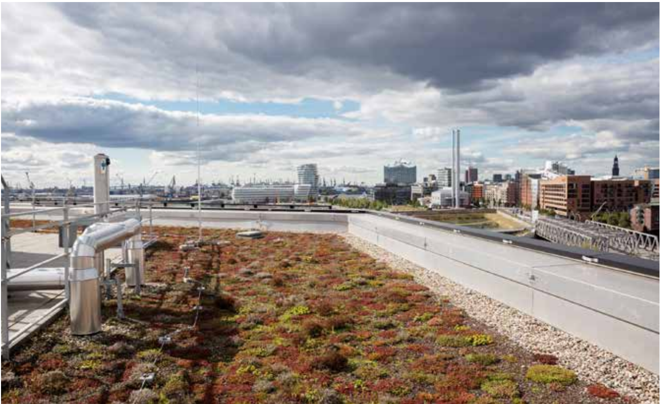
Green roof of HafenCity University Hamburg. Hamburg has started implementing measures to keep the rain water in place or store it, for example through the green roofs program. Photo by Isadora Tast/Hamburg Ministry of Environment and Energy.
