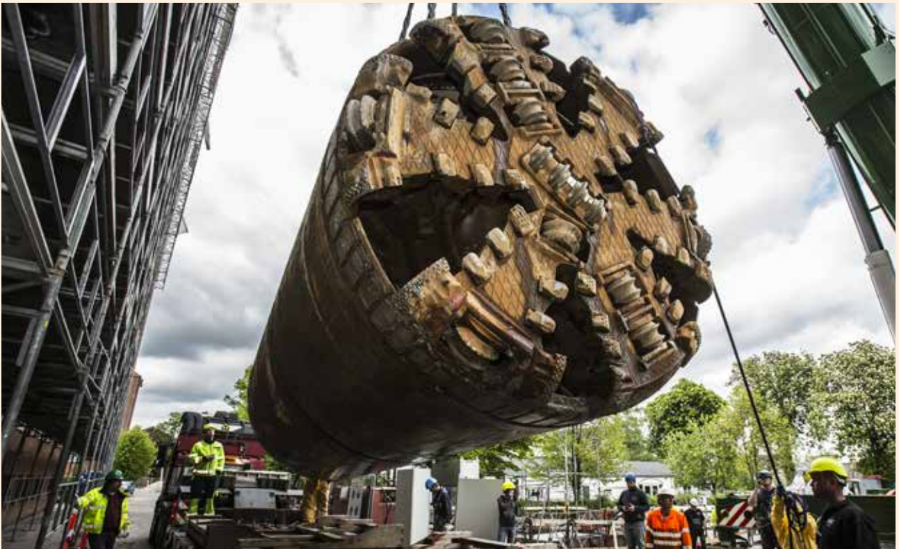
Preparation of the tunnel boring machine for the Østerbro tunnel. The tunnel has considerable hydraulic effect as it will ensure that water from cloudbursts can be safely directed from Østerbro towards the harbour. Photo by HOFOR
