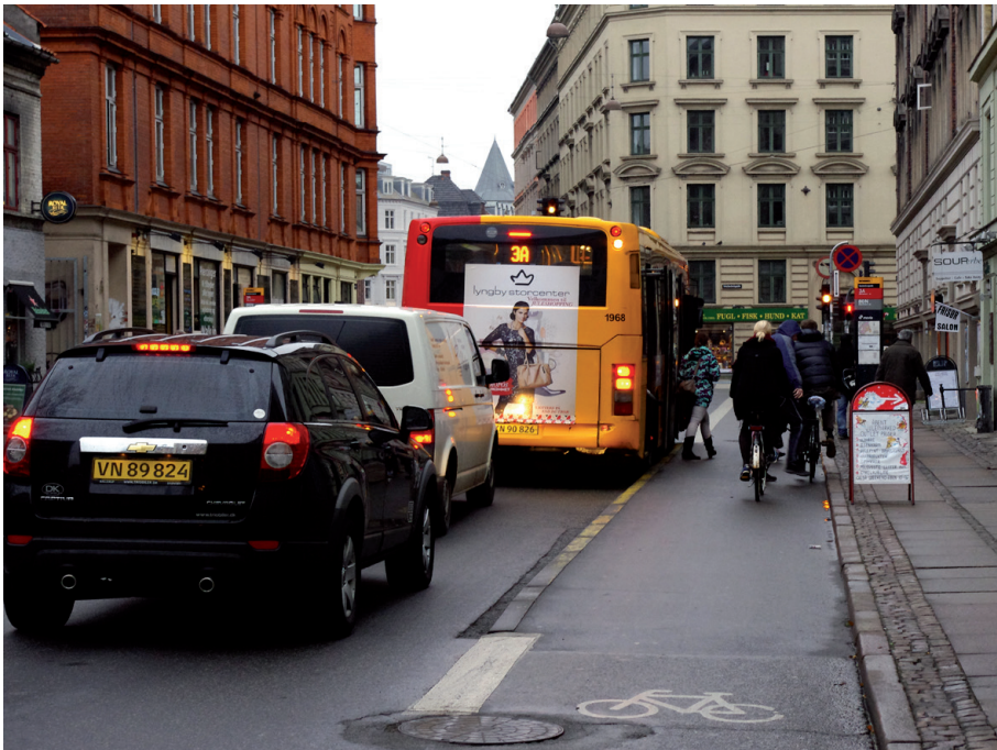
This kerbside bus stop has no passenger platform and a cycle track runs through it; cars must wait for the bus to leave. Enghavevej at Vesterbrogade.
