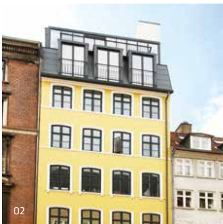
02 Ny Vestergade 3 Tegnestuen B19 / Completed 2013 Ny Vestergade 3 is an apartment building from 1848 that has been renovated and rebuilt. The original building has been preserved, and a new penthouse floor has been added. The new elements interface directly with the old as a contemporary interpretation of the existing architectural character.
